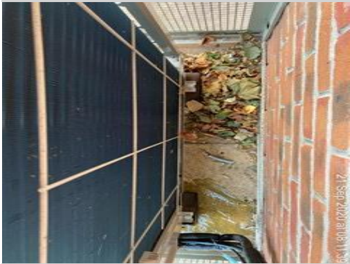
Figure 3 - AC02 Condenser coil clean
