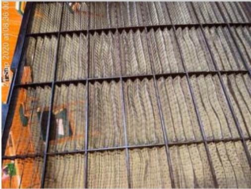
Figure 4 - AC02 Filter clean
