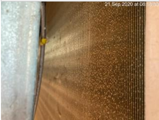
Figure 6 - AC08 Condenser coil clean
