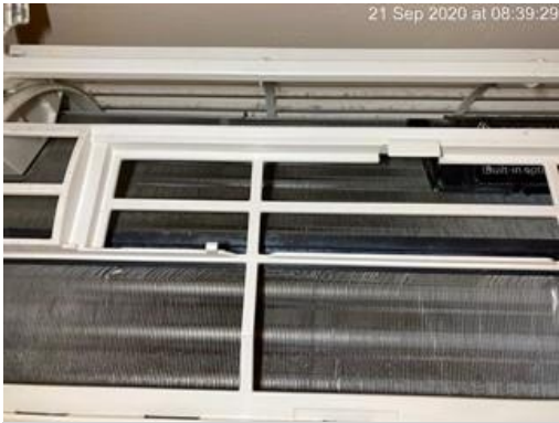
Figure 2 - AC01 Coil clean
